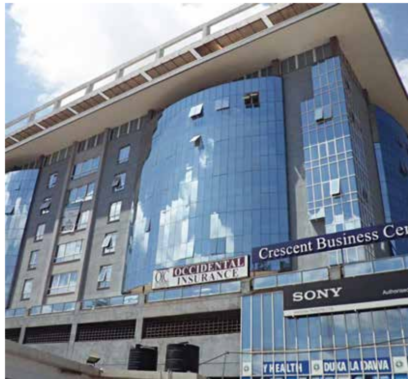
Crescent Business Centre in Nairobi was one of Shyam's first projects as a labour contractor. (NB: Shyam was Main Contractor in all the other projects pictured here.)
