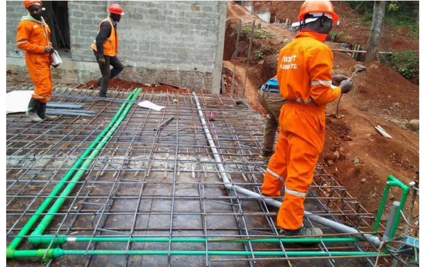
Trident Plumbers Limited on site
