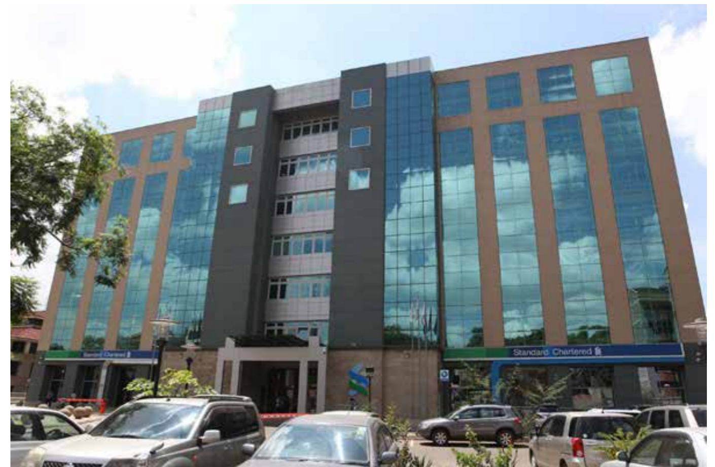
Standard Chartered Bank Headquarters Nairobi (Image: Coolplus Technical Services)
