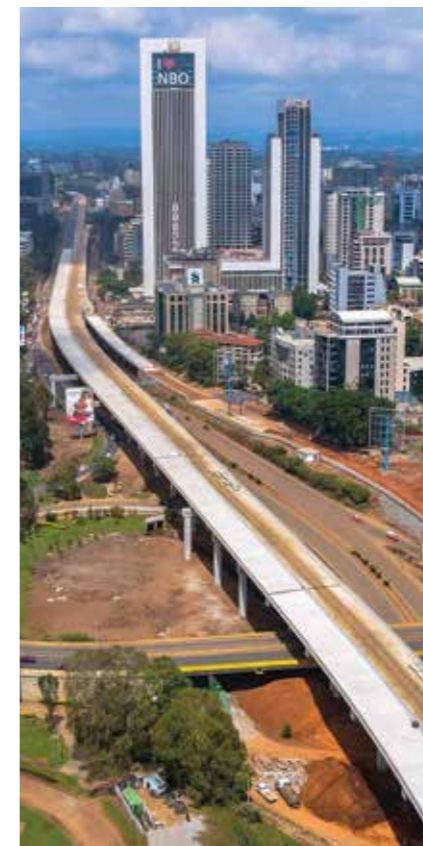
A section of the Nairobi Expressway near the Museum Exit/Entry
