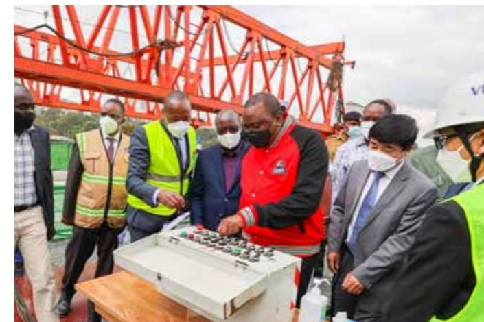
At the end of December 2021, President Uhuru Kenyatta launched the last box girder along the main alignment of the Nairobi Expressway. The project is expected to be complete in March 2022.
