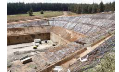
A section of the stalled project
