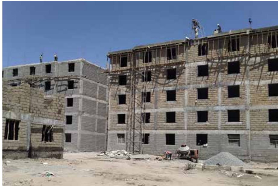
Part of the 605-unit project. (Image: Kenya News Agency)
