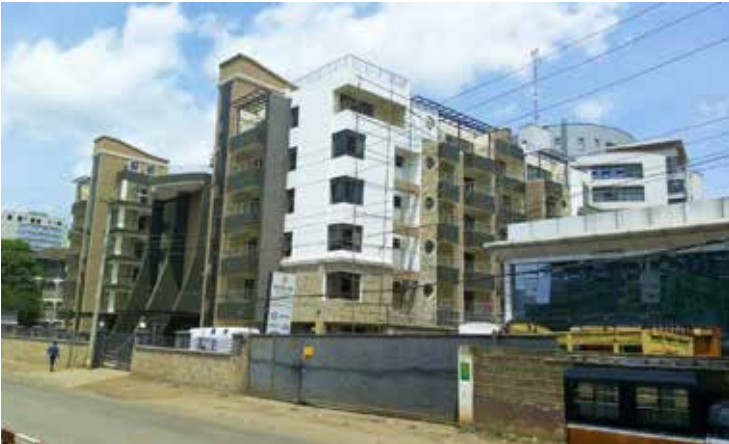
Kenyatta National Hospital Staff Sacco apartments, Westlands
