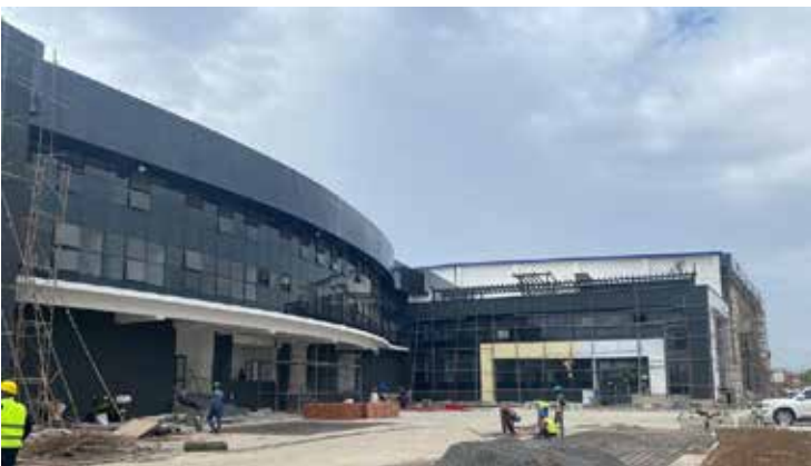
The KEMSA warehouse under construction
