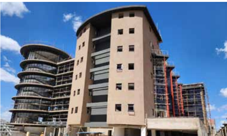
The KEMSA office block under construction
