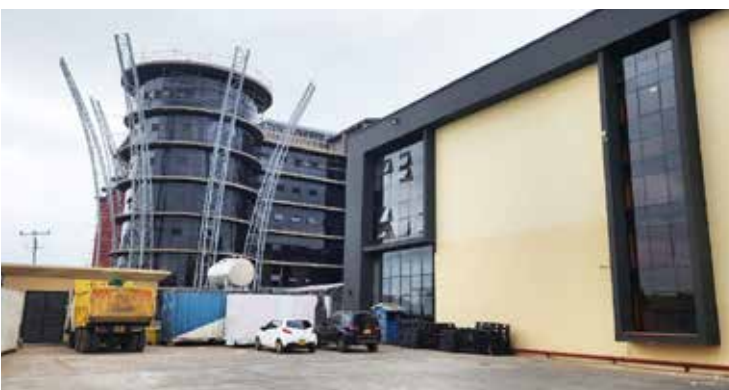
Another view of the KEMSA office block and warehouse
