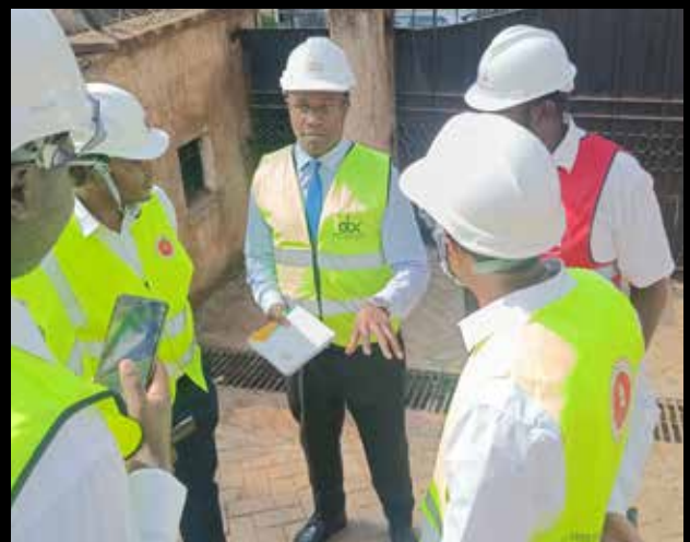
A multi-agency team on a recent routine inspection of a construction site in Nairobi to ensure deep excavation does not interfere with surrounding buildings.
