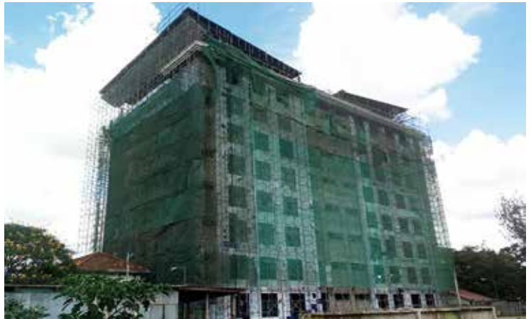
The KICD Headquarters – Phase 1 – Office Block
