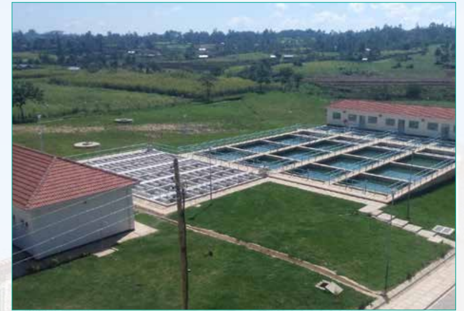
Mumias Water Treatment Plant
