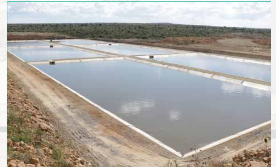
Narok Town Sewerage project
