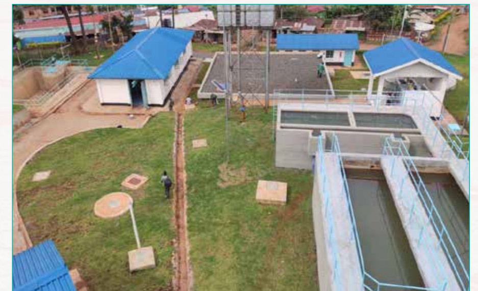
Nyamira Treatment Works
