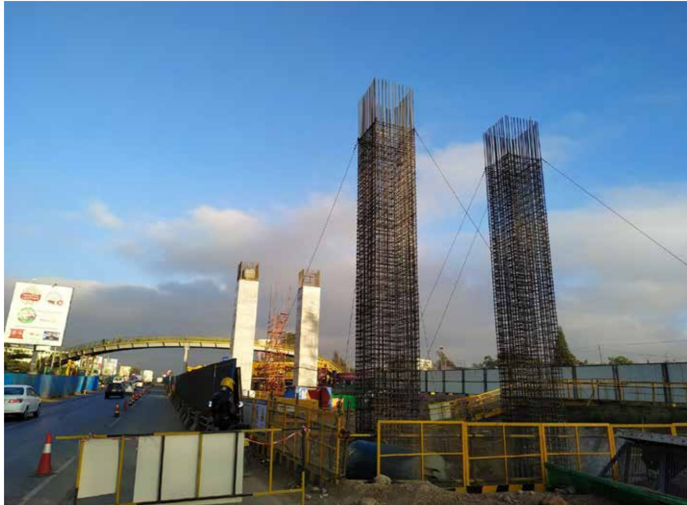
The Nairobi Expressway while under construction.
