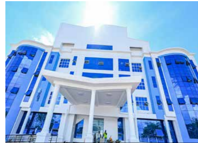
This is the new home of Kisumu Water and Sanitation Company Limited (KIWASCO). Kisumu County Government has accelerated the construction of facilities within the lakeside city.
