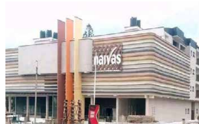
The Catholic Diocese of Kakamega embarked on a mixed-use development project in the heart of Kakamega Town. Overseen by Brickehaus Ltd, the project is racing towards completion.
