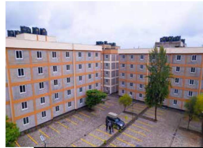
A section of the Ksh 2 billion Bondeni Affordable Housing project in Nakuru. The project was finally completed earlier in the year and is ready for occupation.
